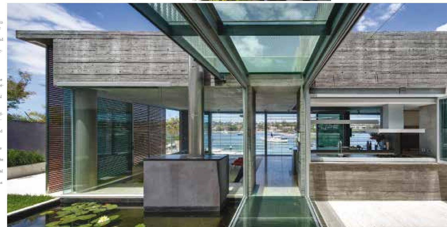
The design incorporates a number of passive climate control measures such as thermal mass in the concrete slabs and walls; a 10,000-liter rainwater tank; and a garden roof which further insulates the building below and reduces storm water run-off. Deep overhangs and retractable blinds reduce the summer heat gain, while the impact of cross ventilation is amplified by reducing the building depth by the central courtyard and using bodies of water adjacent living spaces as cooling elements.
