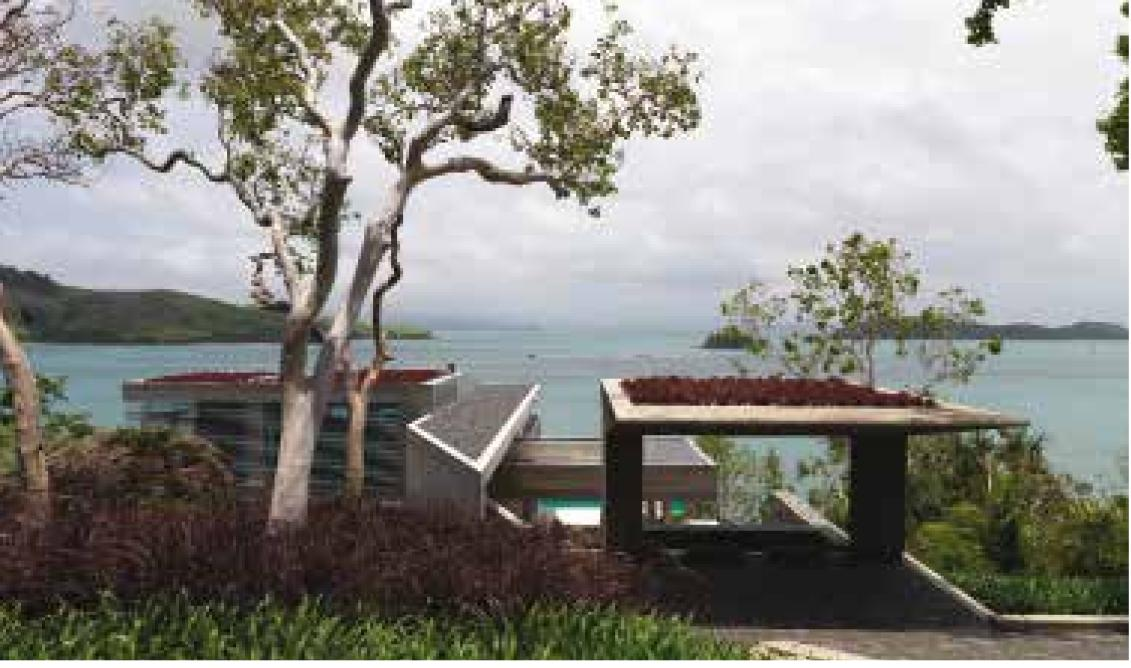
The architecture incorporates a number of passive climate controls, such as deep overhangs that shade the interior, massive concrete walls or green roofs. Combining architectural energy-saving design principles along with material selection removes the need for other finishing trades and materials, requiring very little on-going maintenance, staying resilient to the extreme weather conditions of the tropics and avoiding regular repair and replacement maximizing the building's life span.
